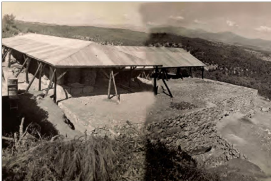
Figure 4.19 Temporary wavy sheet roof (Source: Çambel,2010, p:134)
