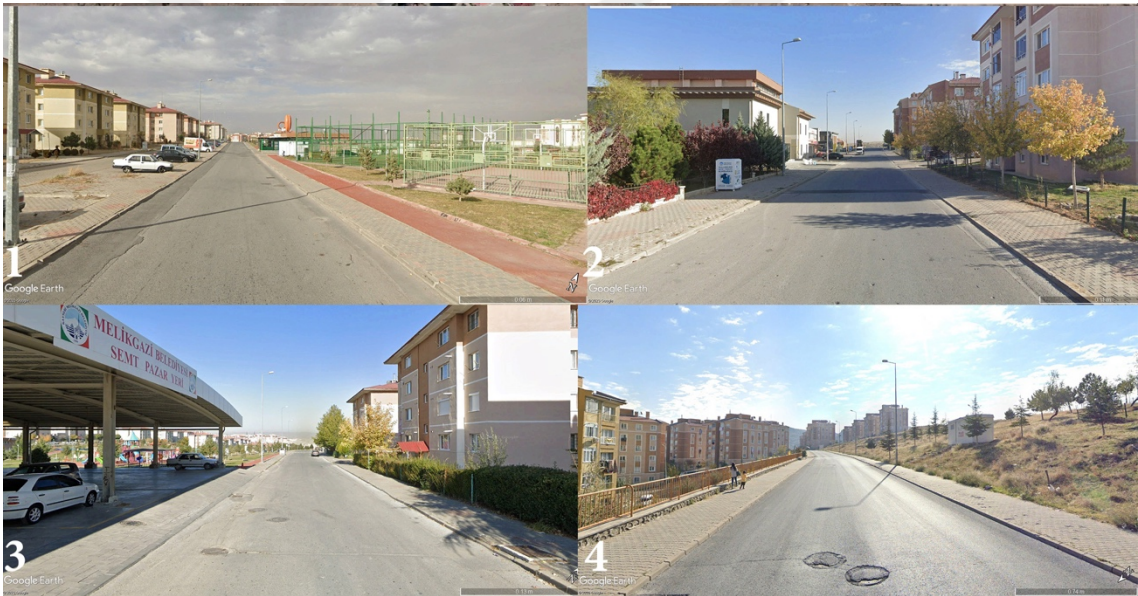
Figure 4.1.9 TOKİ 1-TOKİ 2 street images (Source: Prepared by the author based on Google Earth street images, 2023, Google Earth )
