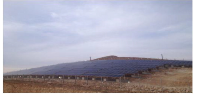
Fig. 1. 250 kW PV plant site.
