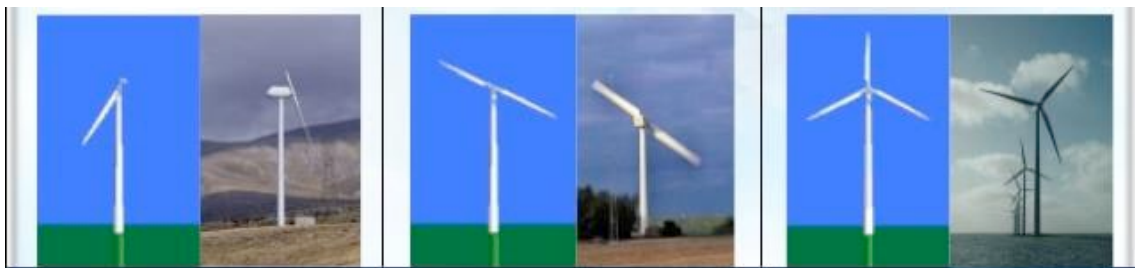
Figure 2. 3 Single-blade, double-blade and multi-blade turbine (www.dolcera.com/wiki/index.php?title=Different_Types_and_Parts_of_Horizontal_Axis_Wind_Turbines)
