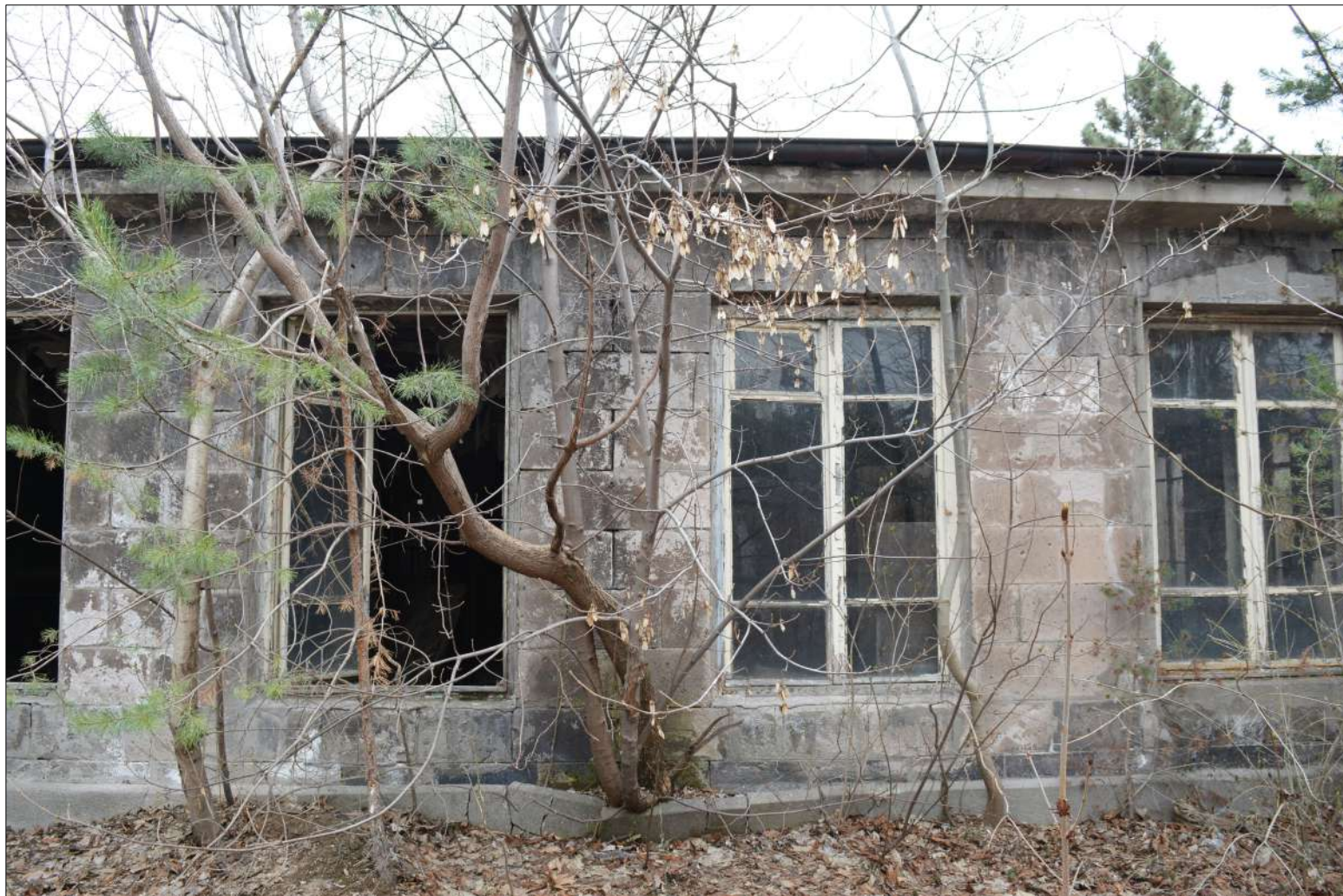
Figure 4.30 Western section of the north façade
