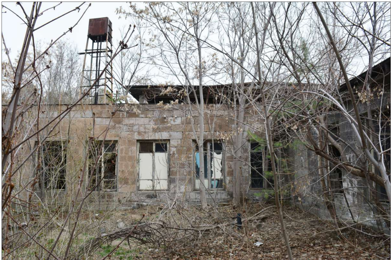
Figure 4.24 Northern section of the western façade
