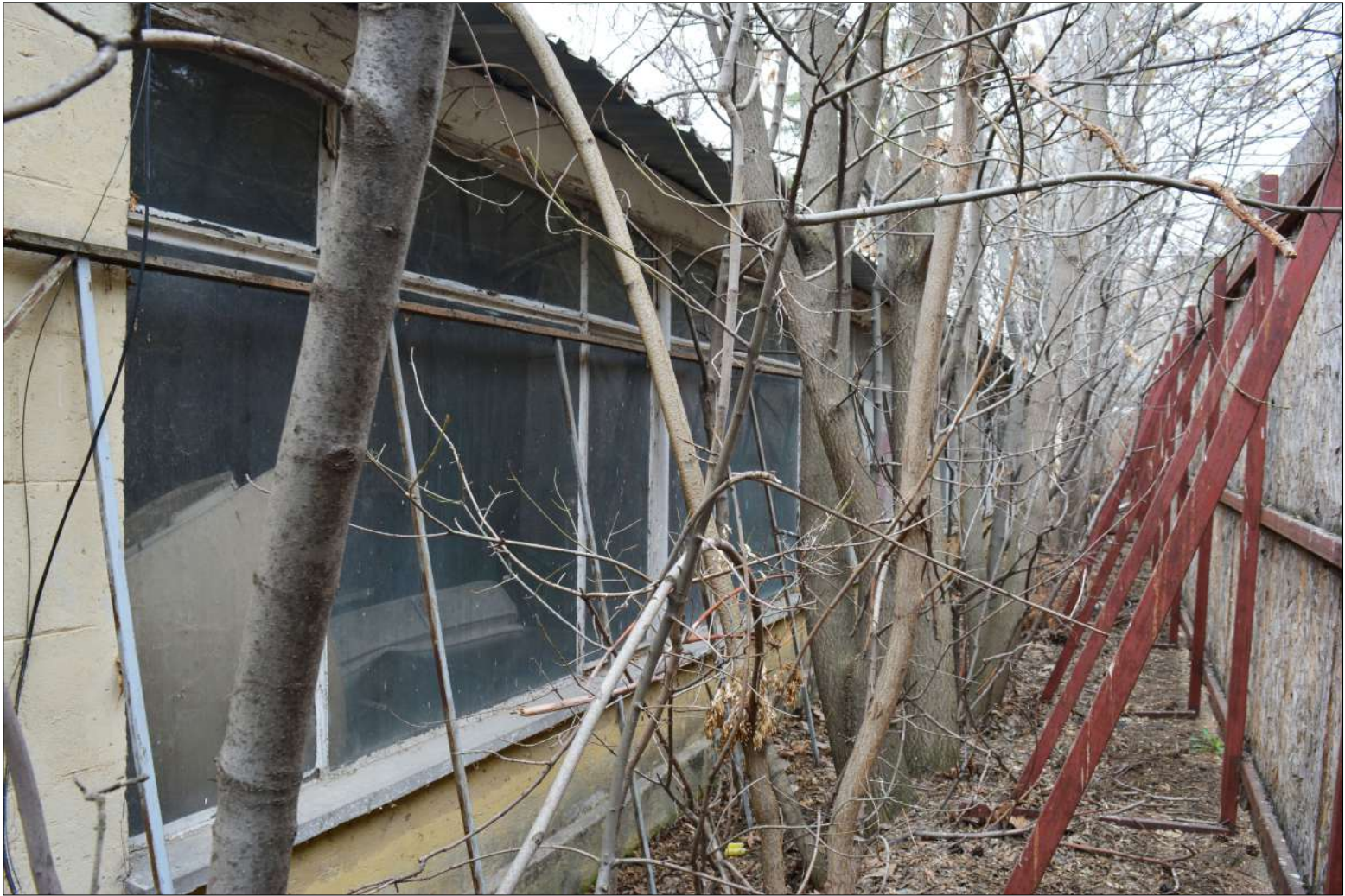
Figure 4.22 View of the foyer section of east façade
