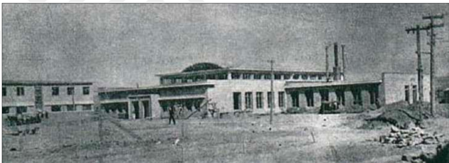
Figure 3.7 Construction of the Employees' Club Building (Eren, 2019)
