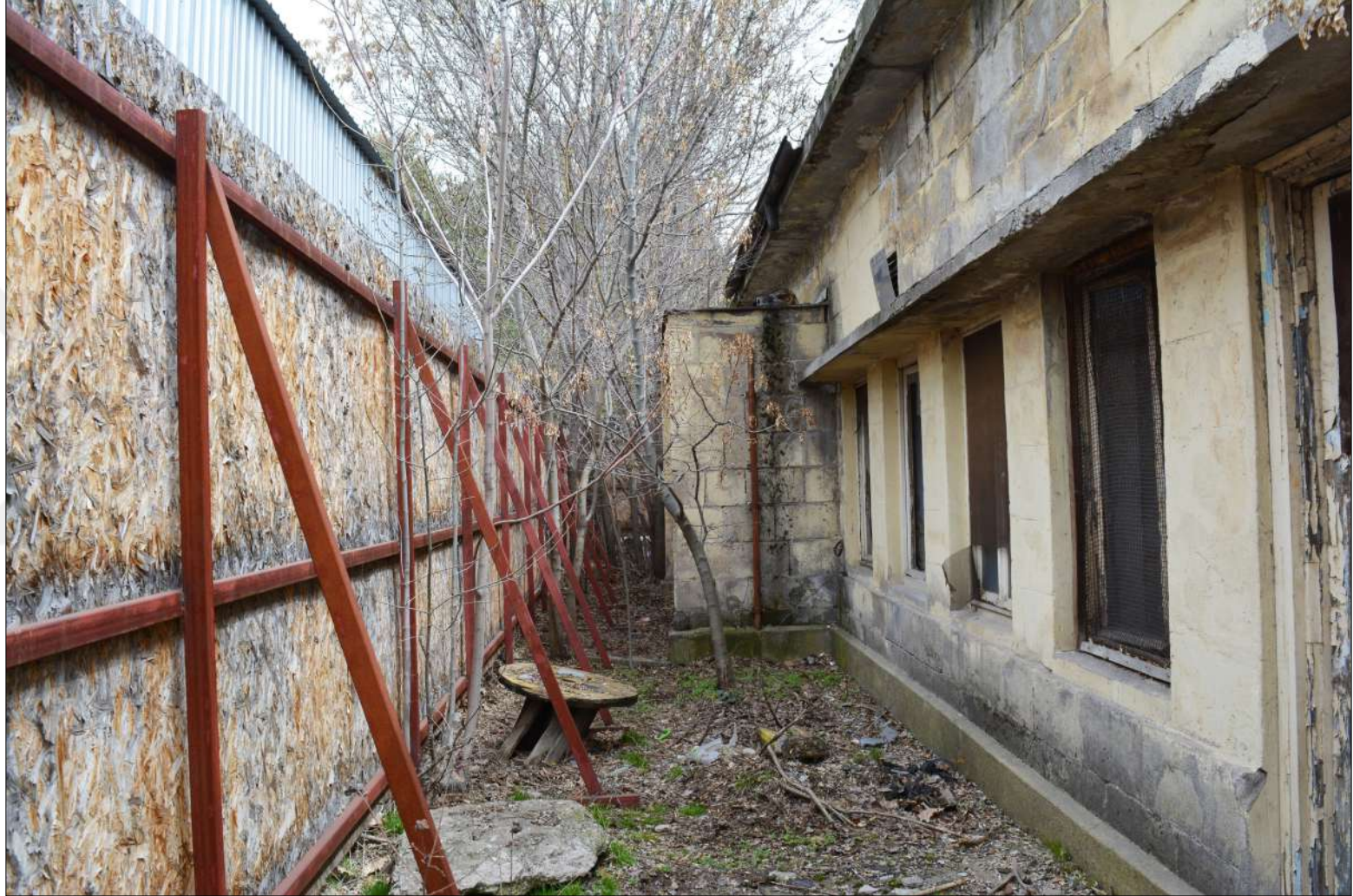
Figure 4.29 Eastern section of the north façade
