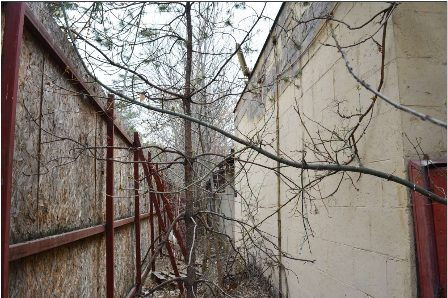
Figure 4.23 Northern section of the east façade
