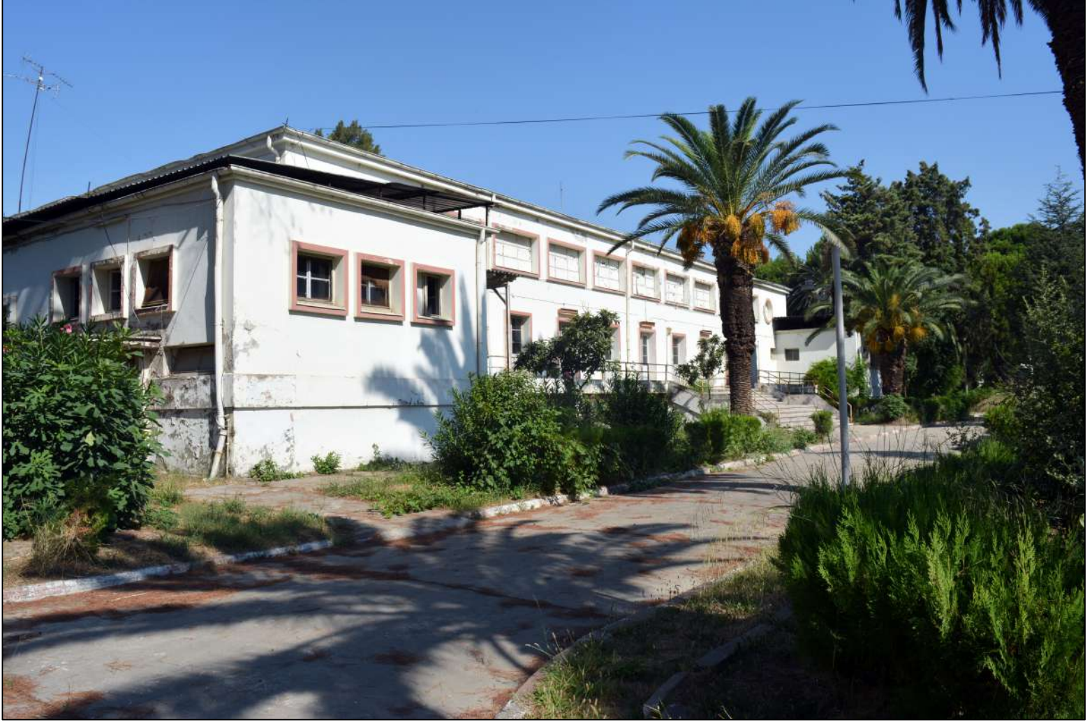
Figure 2.6 Sümerbank Nazilli Printed Factory, Club Building (Source: It was taken by the thesis author during the fieldwork in July, 2022)
