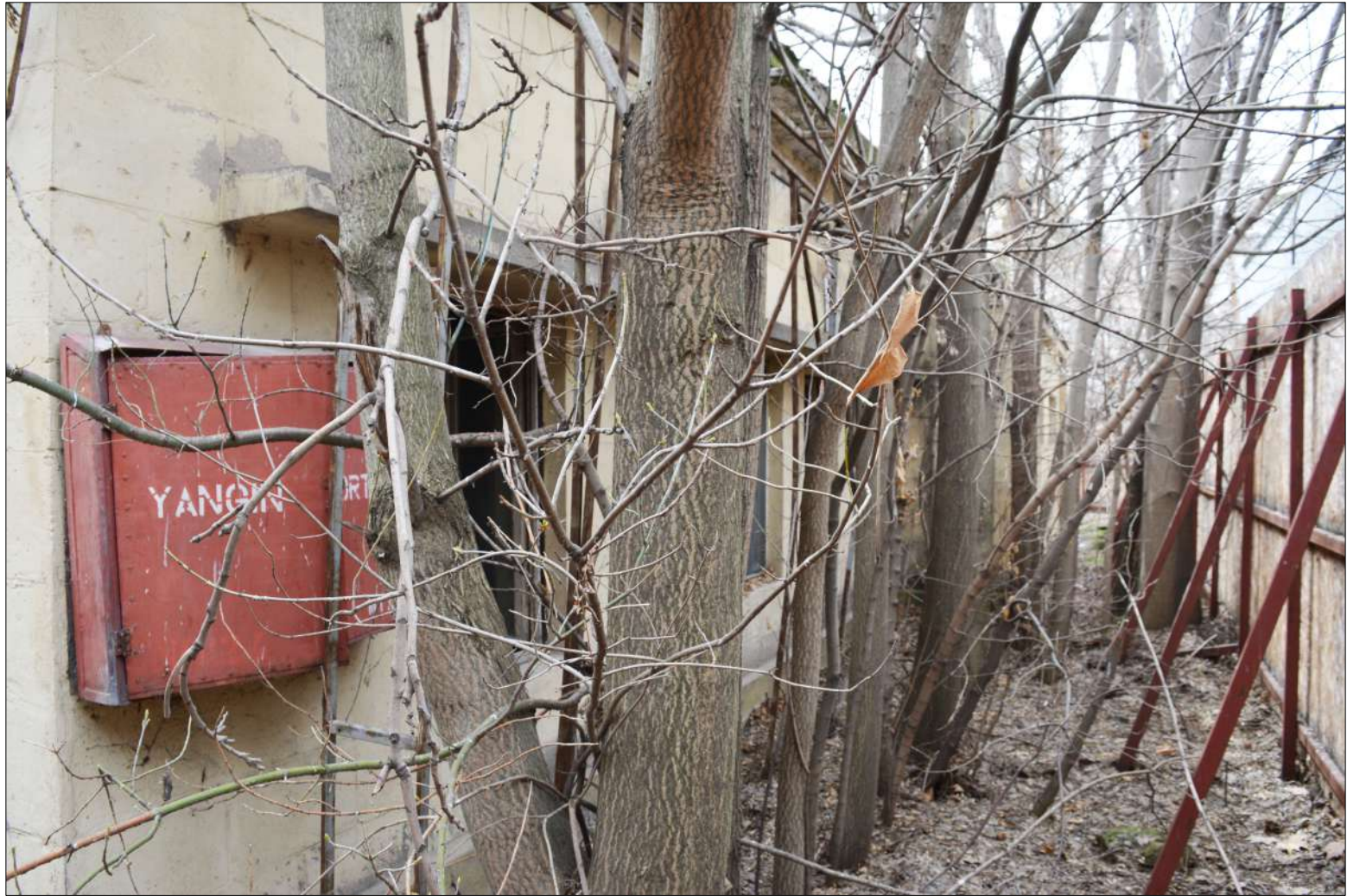
Figure 4.28 Eastern section of the north façade
