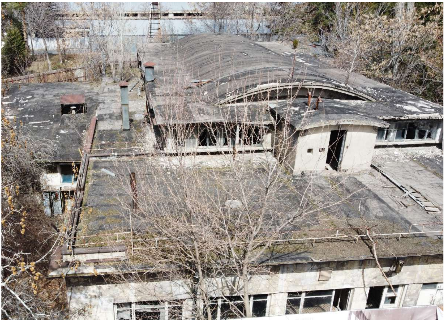
Figure 4.35 View of the roof
