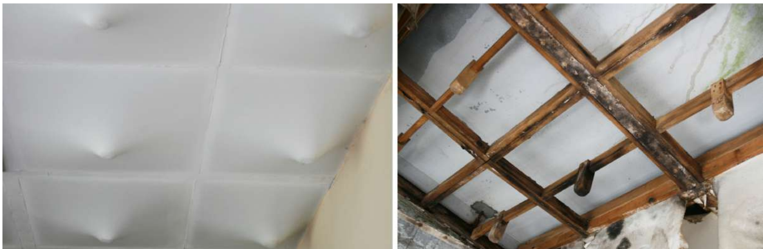
Figure 4.33 Wooden suspended ceiling
