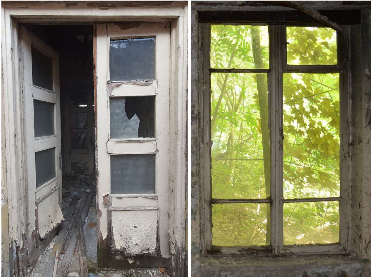
Figure 4.31 Entrance door (D42) and wooden window (W20)
