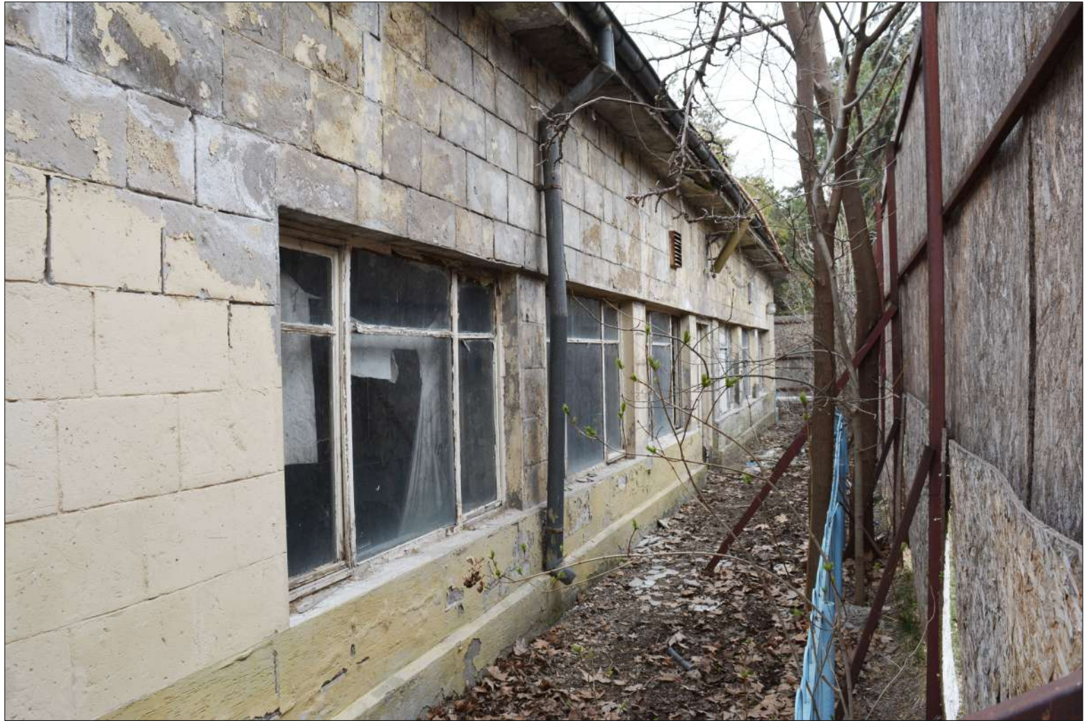
Figure 4.27 Eastern section of the south façade
