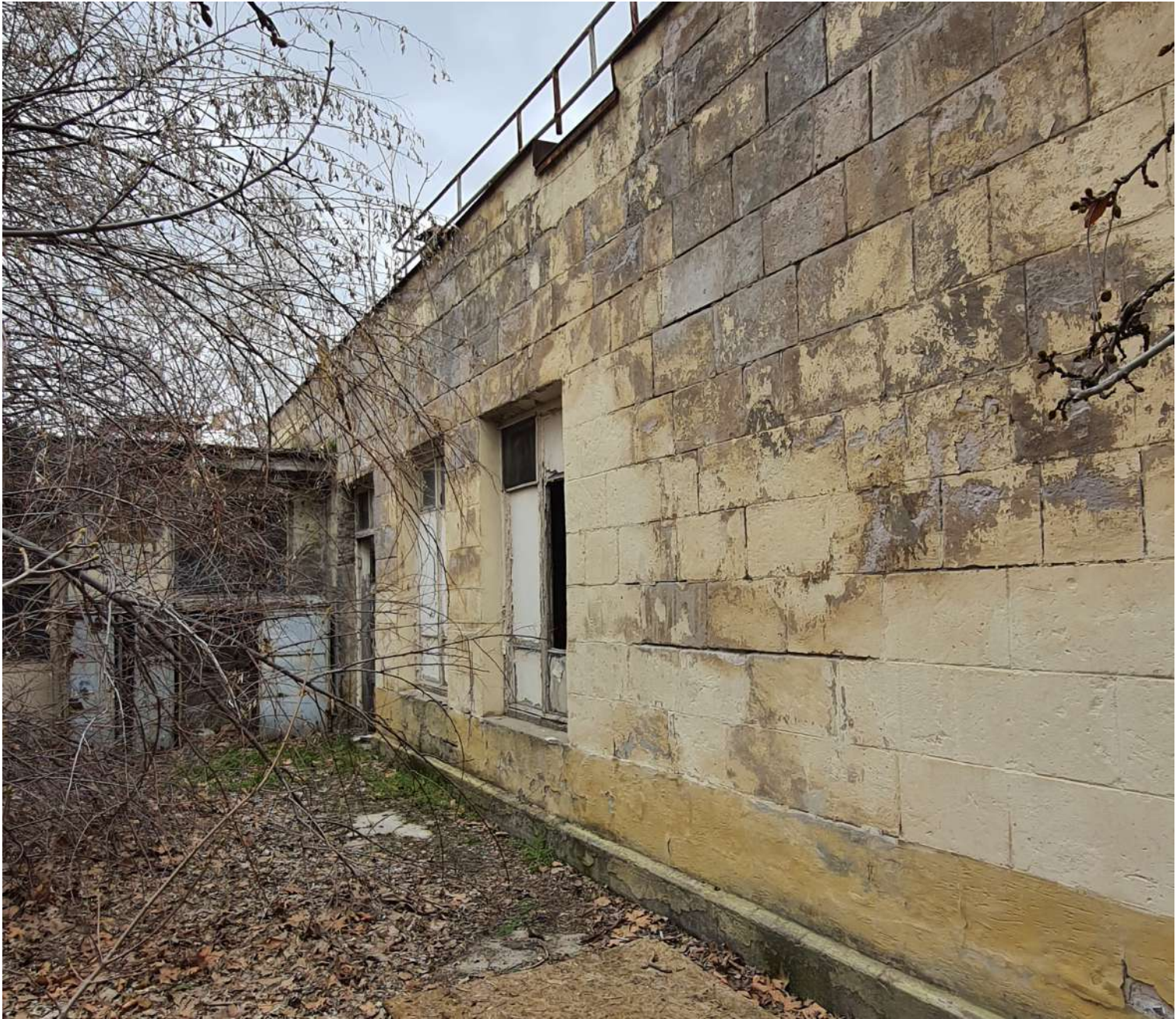
Figure 4.26 View of the southern section of the western façade
