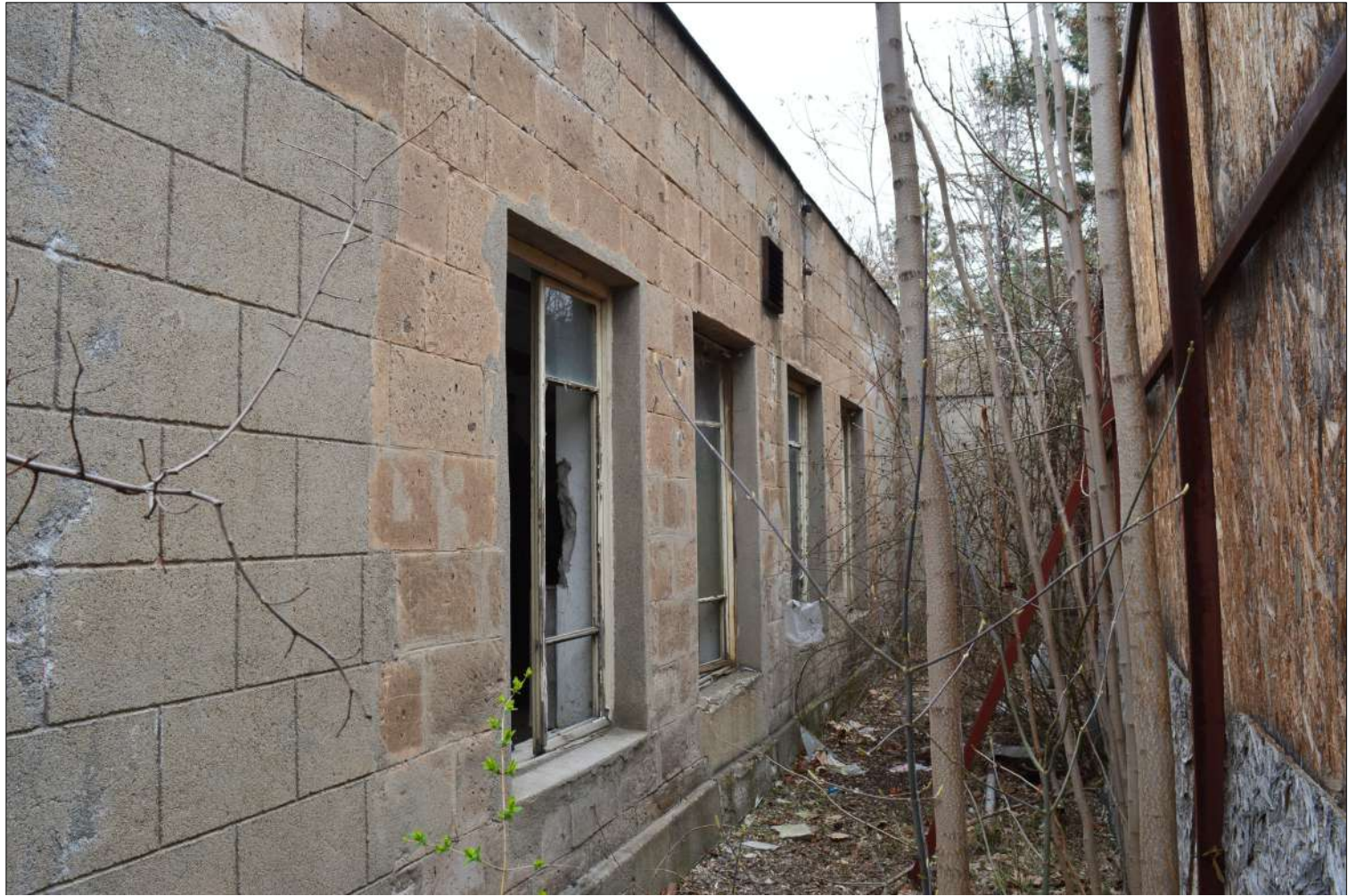
Figure 4.25 View of the protruding section of the western façade
