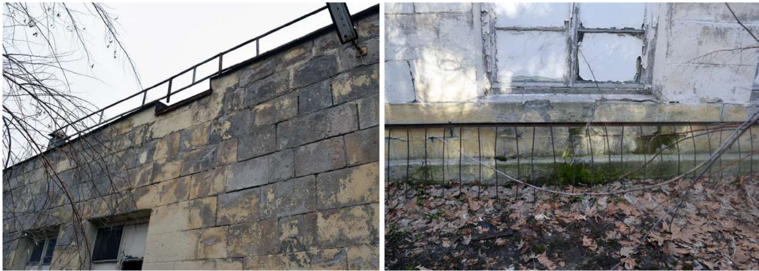
Figure 5.4 Traces of the access to the upper level
