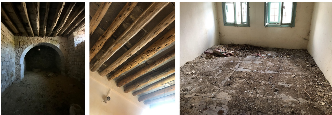
Figure 5.71 Authentic ceiling and flooring
