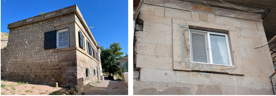
Figure 5.77 Changed window frames
