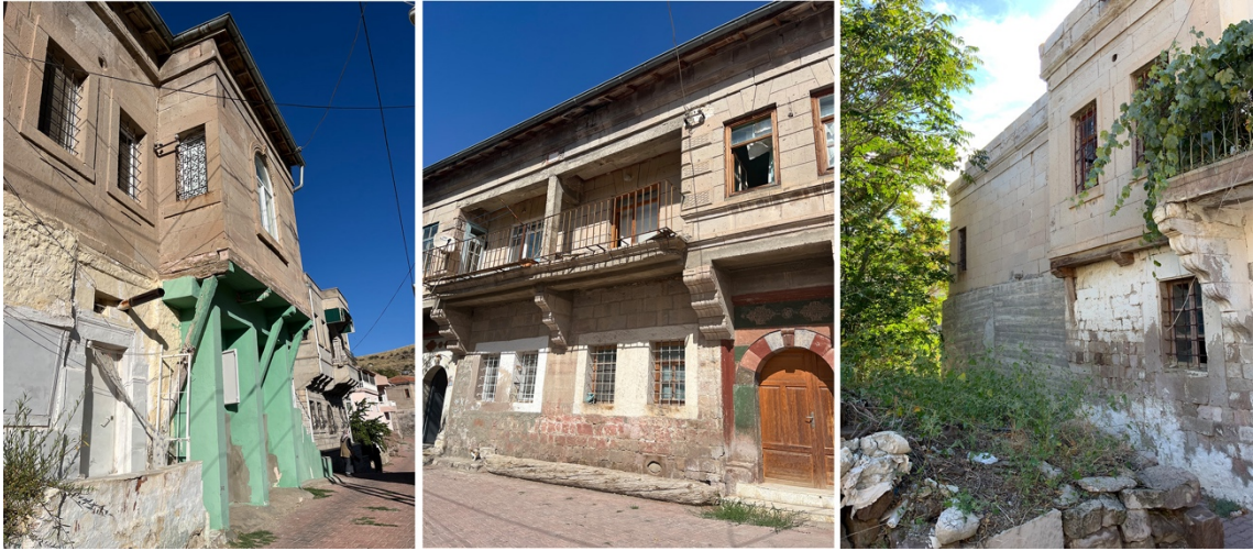
Figure 5.66 Reinforced concrete adding to the structural system
