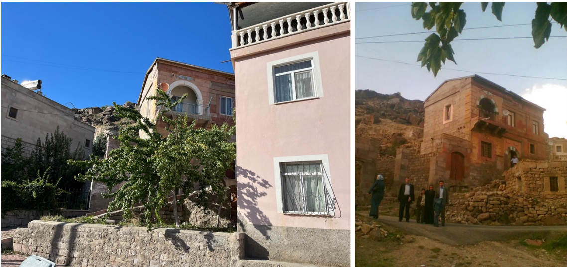
Figure 5.102 Constructed new houses
