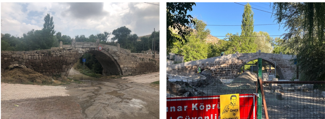
Figure 5.23 Stone Upper Bridge in 2020 (left) and during restoration in 2022
