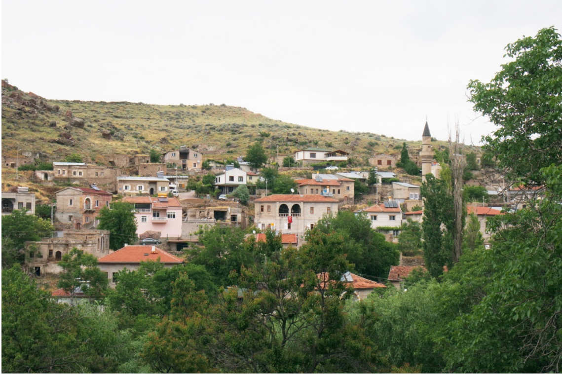
Figure 5.79 New addition pitched roof systems
