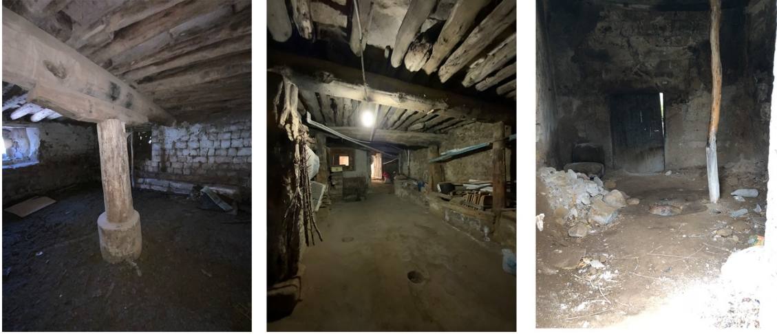
Figure 5.38 Barns at ground floor
