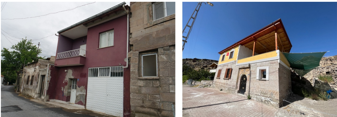
Figure 5.74 Exterior wall interventions
