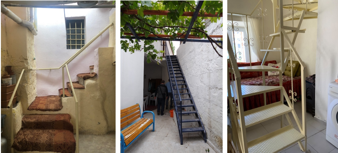
Figure 5.75 New addition stairs
