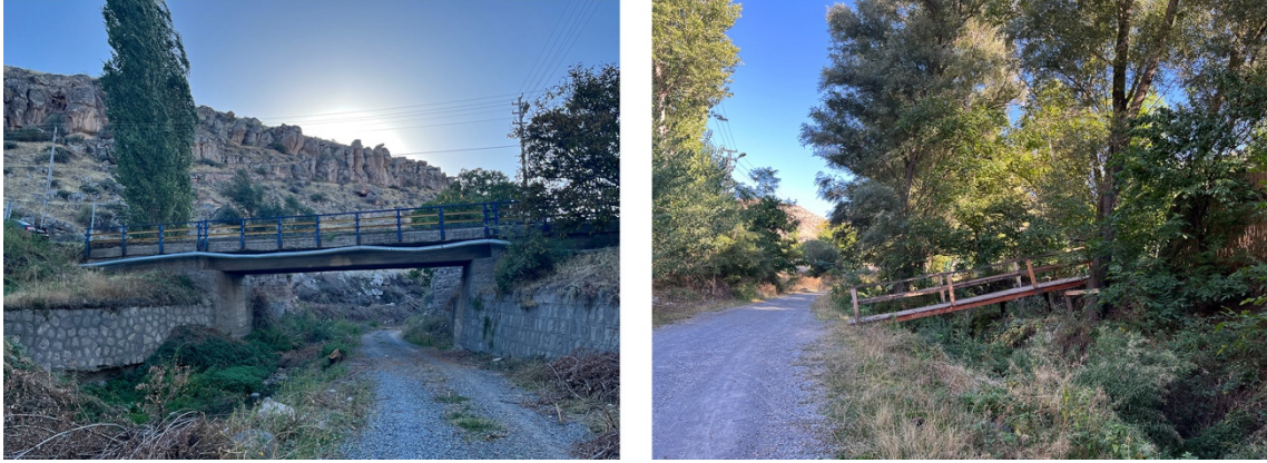
Figure 5.24 New reinforced concrete Lower Bridge and a wooden bridge for passing the stream
