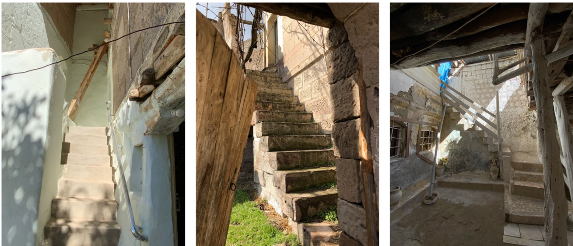
Figure 5.37 Stair types of Bağpınar traditional architecture
