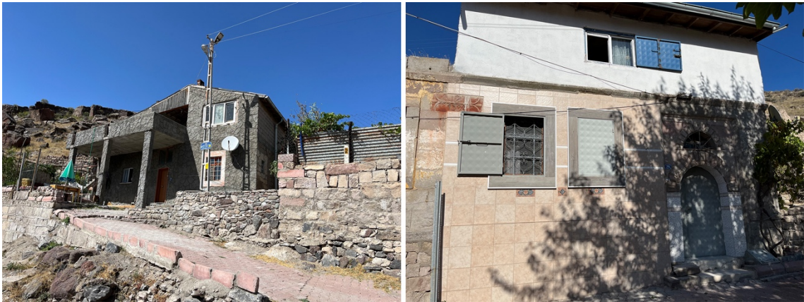
Figure 5.73 Exterior wall interventions
