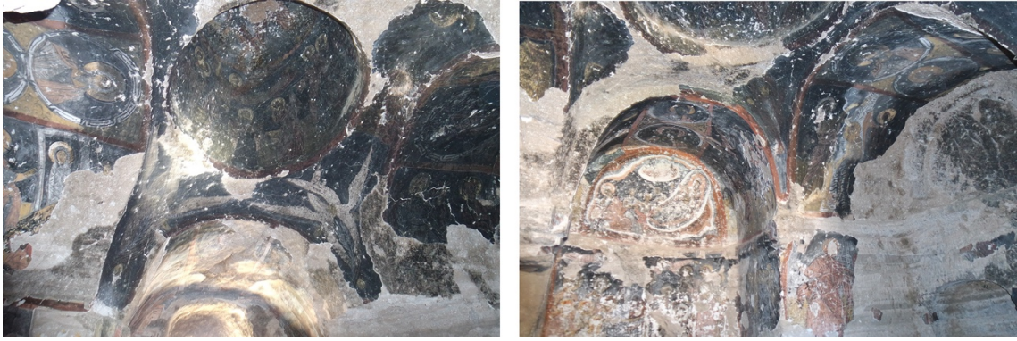
Figure 5.30 Dome and apse of the church
