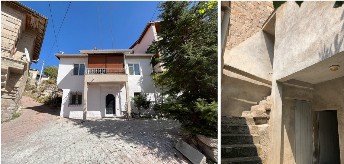
Figure 5.67 Reinforced concrete adding to the structural system
