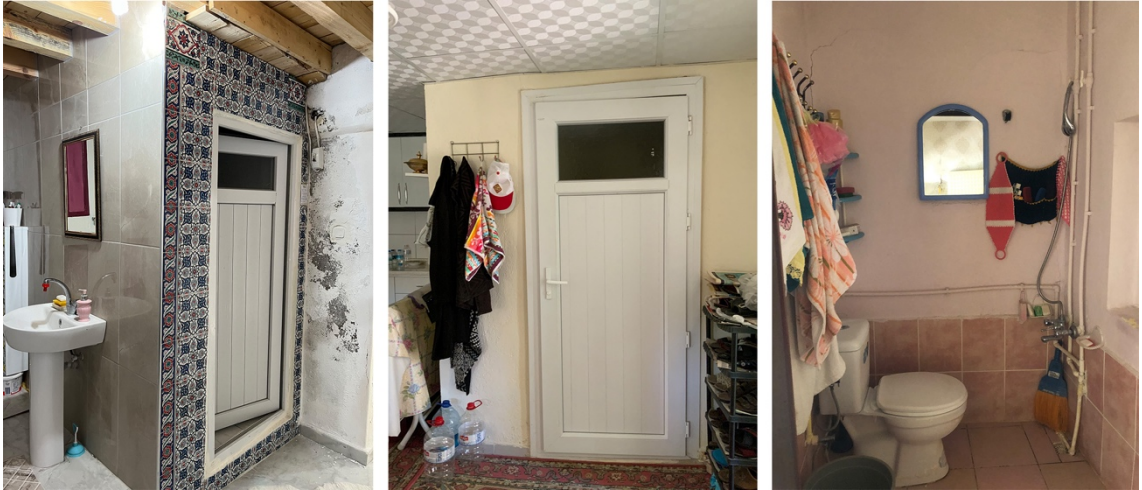
Figure 5.84 New addition wet spaces
