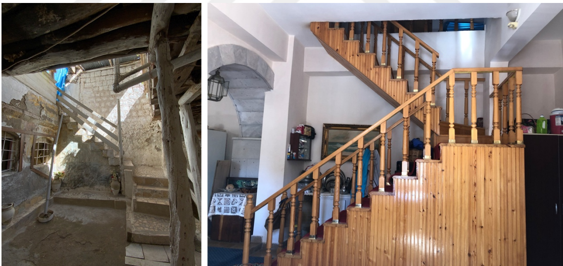
Figure 5.76 New addition stairs
