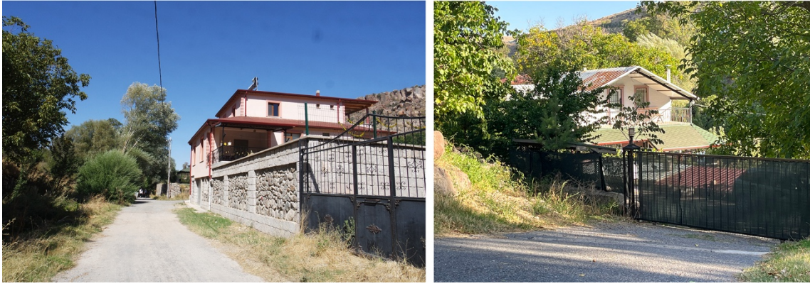
Figure 5.101 New reinforced concrete houses are in the valley bottom
